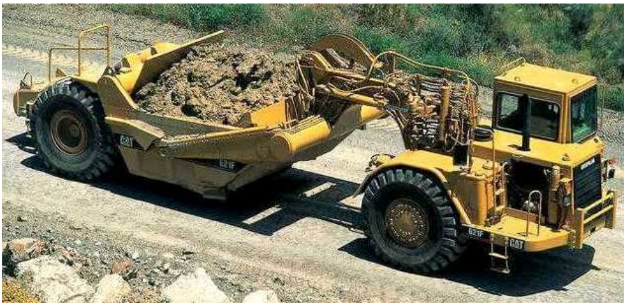
Hauling excavated soil
