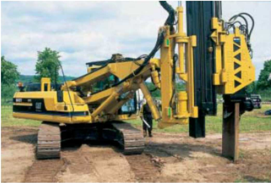
Sheet-wall piling equipment
