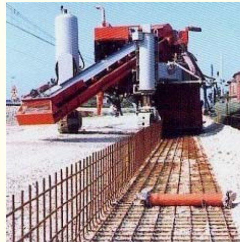
Kerb (curb) construction by concrete finisher
