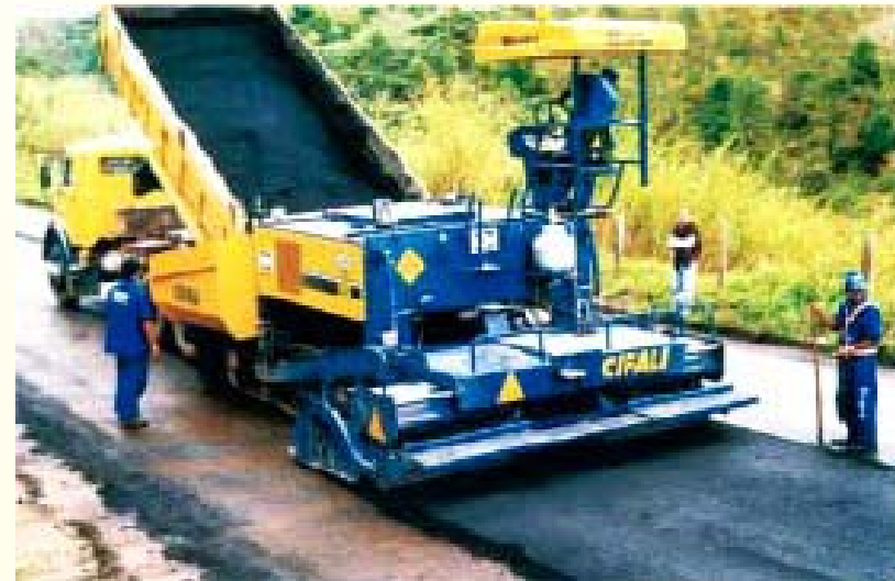
Asphalt finisher in action
