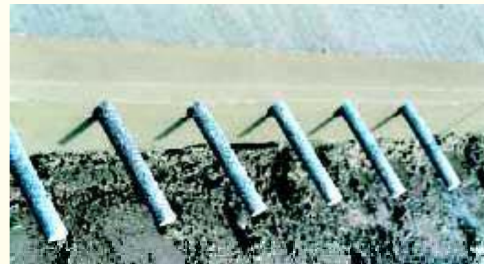
Transversal joint-bars inserted (for joining parallel lanes)
