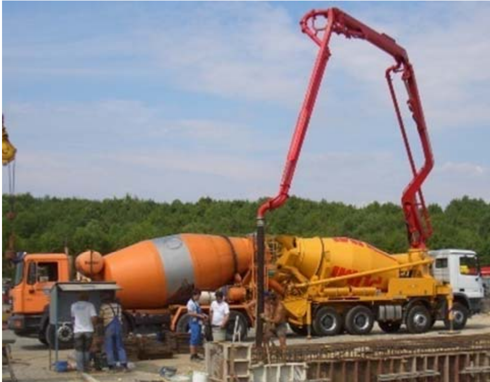
Mixer truck and "pumix" co-operating at the site
