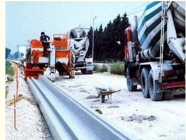
Kerb (curb) construction by concrete finisher
