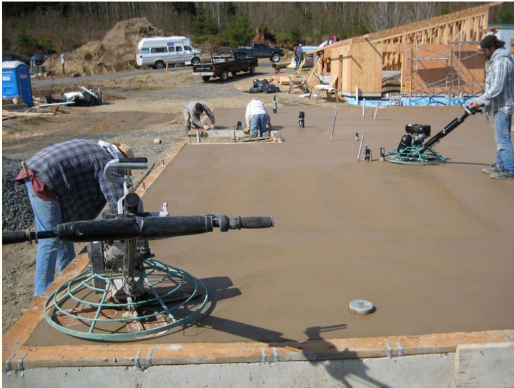
Power trowels in action
