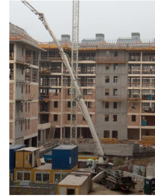
with concreting pump
