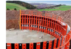
circular wall formworks
