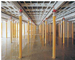
panelized slab drophead formwork system
