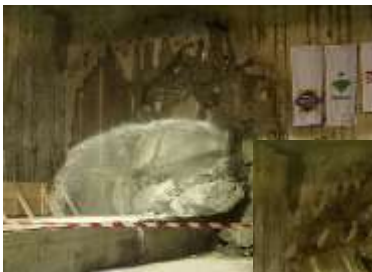
TBM arrives to Bocskai út
