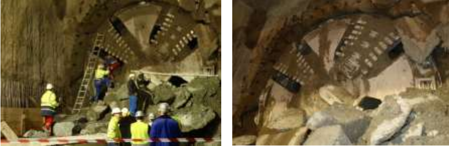
TBM arrives to Bocskai út
