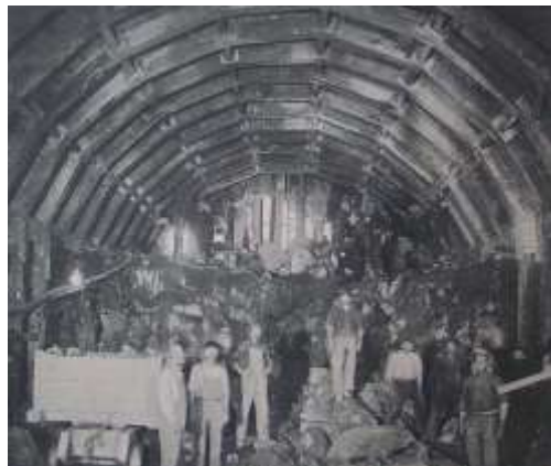
Construction of Fort George Tunnel
