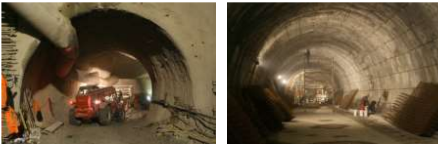
The New Austrian tunnelling method in Budapest
