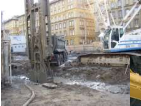
Construction equipment Baross tér
