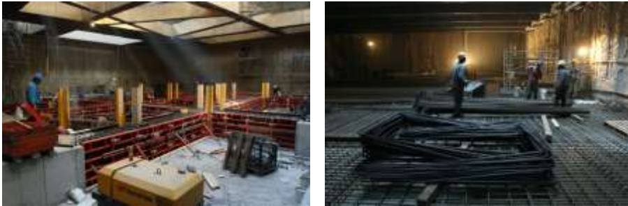
Construction of metro stations in Budapest
