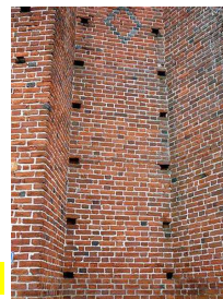
restrained console scaffolding
