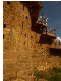
restrained console scaffolding
